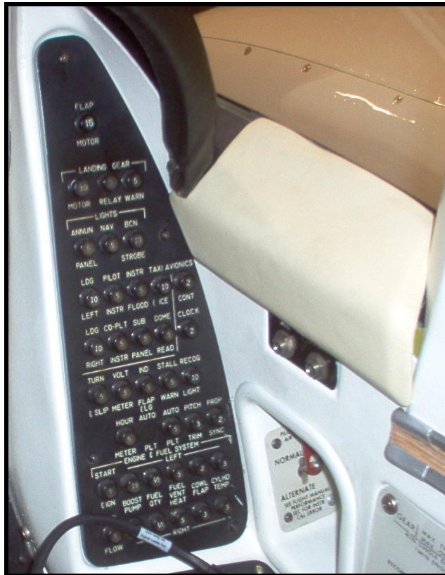
Figure 2: Cowl Flap Circuit Breakers - Engine & Fuel System - Row 8 & 9, Photo by Robert Hoffman
