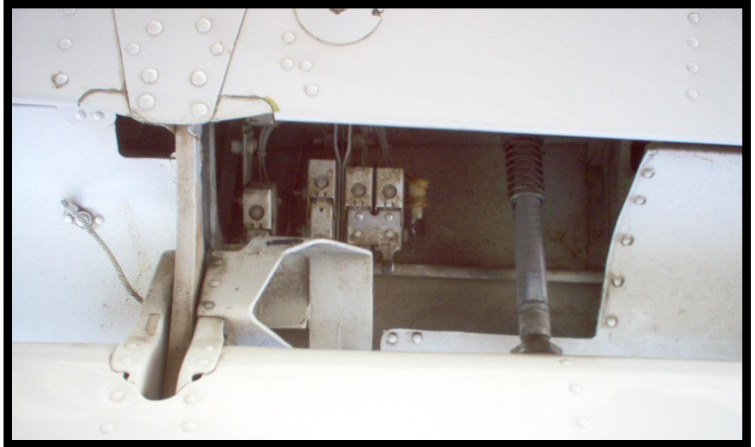
Figure 4. B60 Flap Limit Switches, Photo by Robert Hoffman
