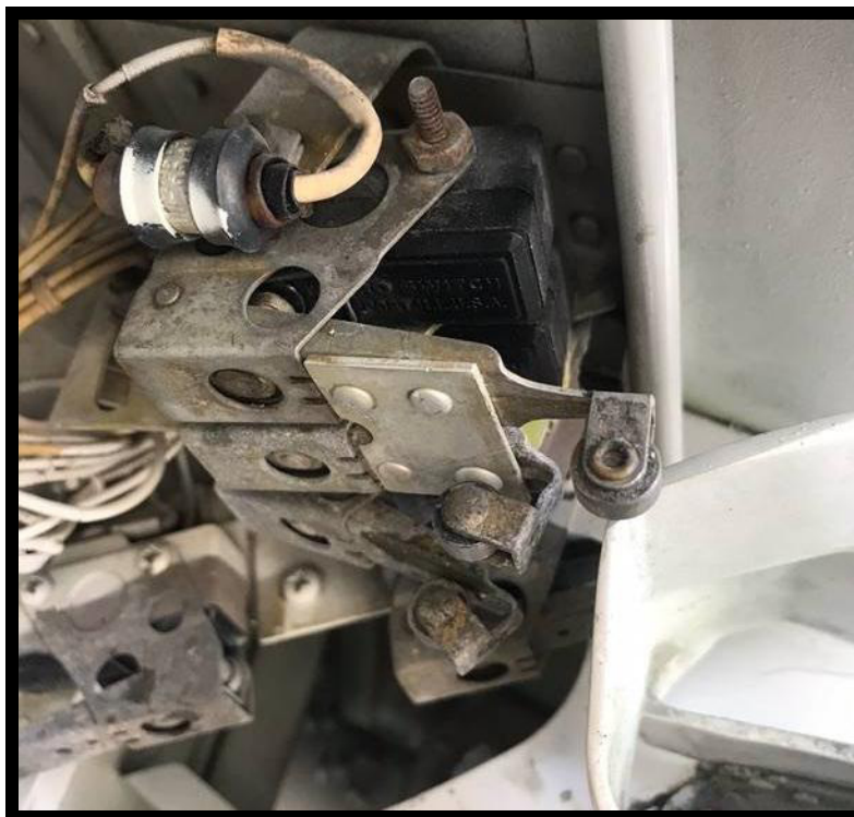
Figure 10. Failed 16 degree limit switches. Photo by Robert Hoffman
